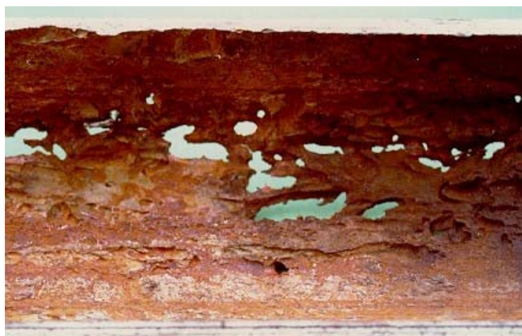
FIGURE 1 - Penetrating localized attack in Oil well 5.
